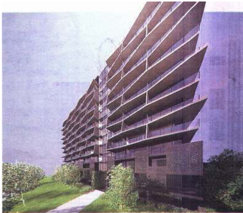
Higher and higher: a multi-storey building will have 156 apartments.
